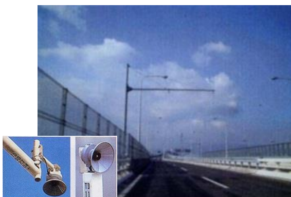
Vehicle Detector (Ultrasonic Detector)
