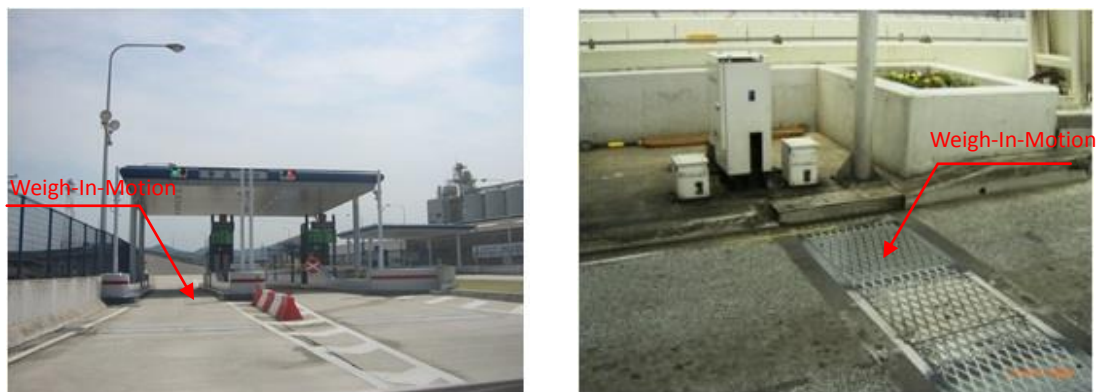
Overload Monitoring System
